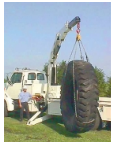
LIFT MADE IN VERTICAL POSITION
