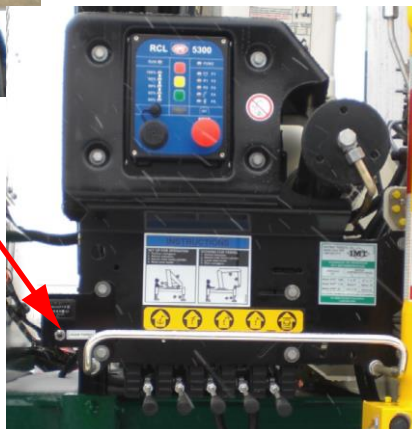
Crane power switch
