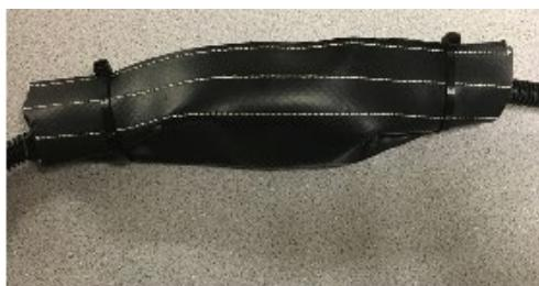
*Step 3: Securely zip tie both ends of the protective sleeve.*
